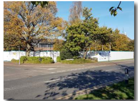
The white boards surrounding the refurbishment works at GE in the centre of the village
